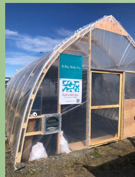
Figure 1 - High Tunnel Installation 2022 (1)
