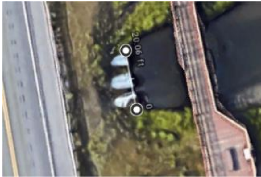
Figure B.5: Measurement of the Culverts
