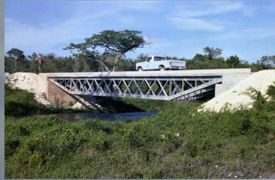
Alternative Two - Steel Under Truss Bridge
