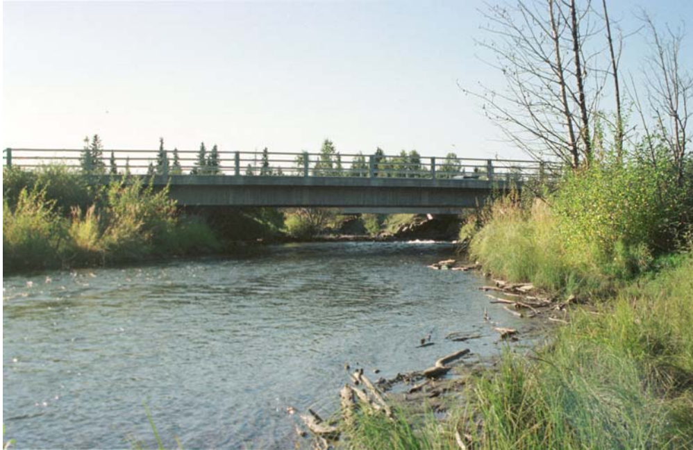
Existing view of Campbell Creek from Campbell Creek Greenbelt, looking west (before project construction)
