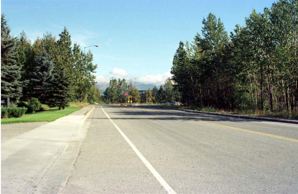
Existing view of International Airport Road, looking east (before project construction)
