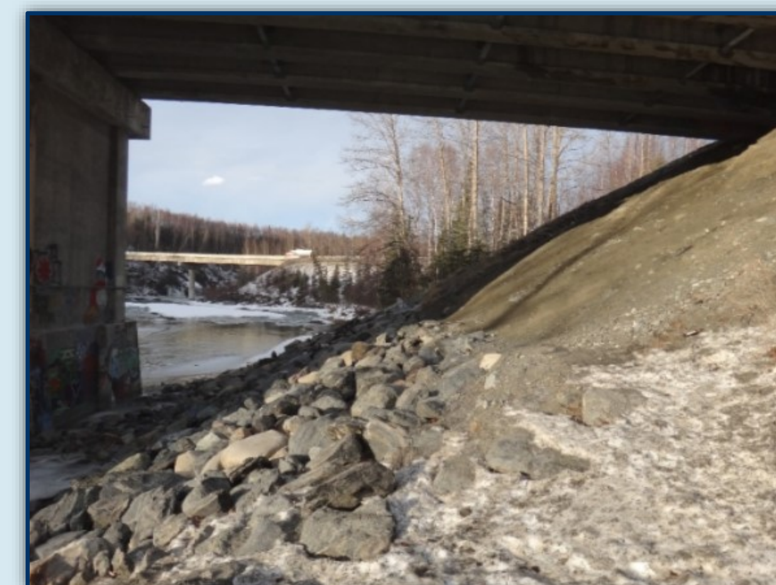
Riprap Along Existing NB Eagle River Bridge
