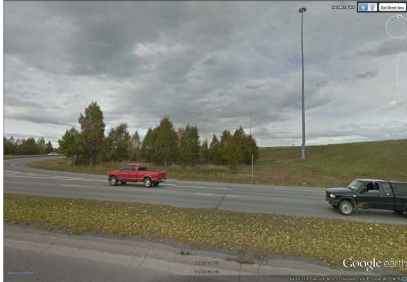
Figure 5: Existing high mast lighting
