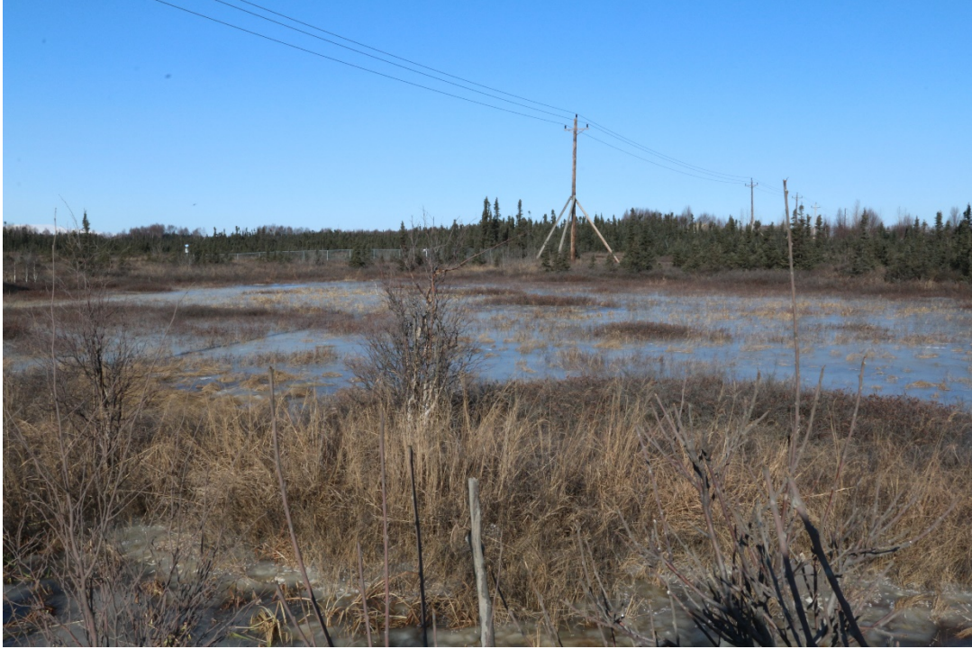
Figure 2: Connors Bog, overhead wires. A photo taken facing north at Northwood and Raspberry of existing overhead facilities
