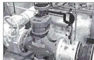
In-line Grinders are Typically Installed on the Suction Side of a Pump
