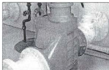
4-HYDRO-I Installed into Pipeline
