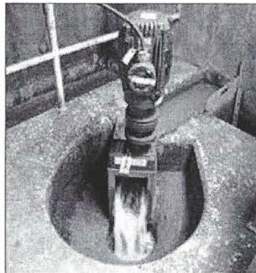
Wet Application 3-HYDRO-C
