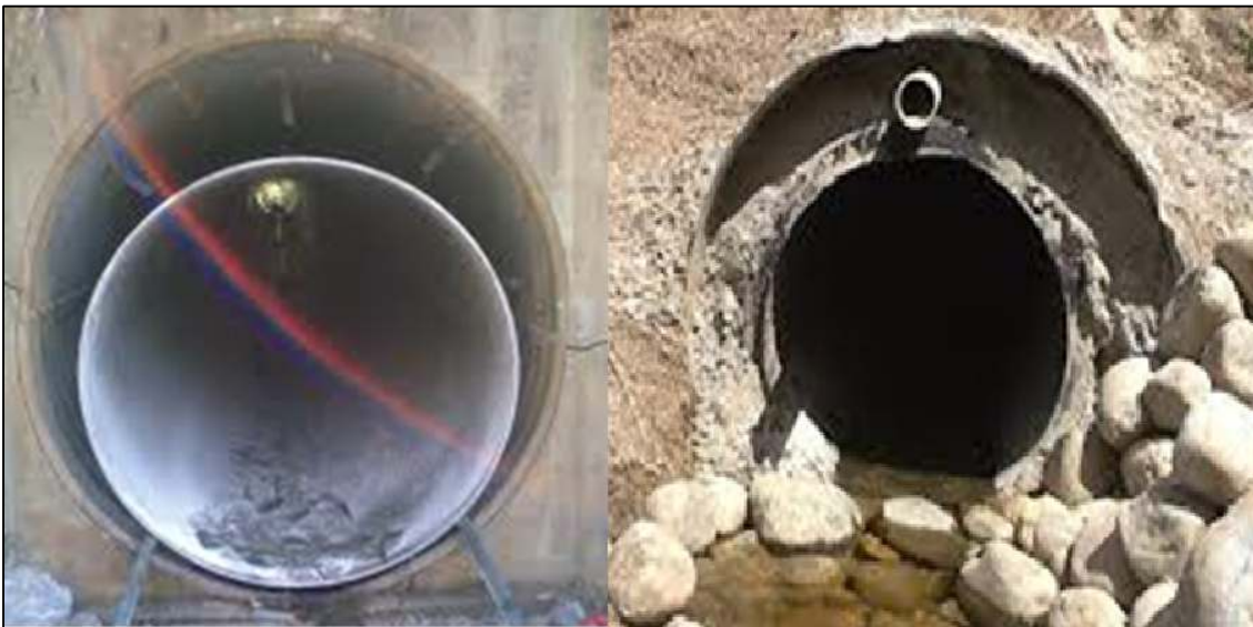
Figure 6: Slip lining – before (L) and after (R)
