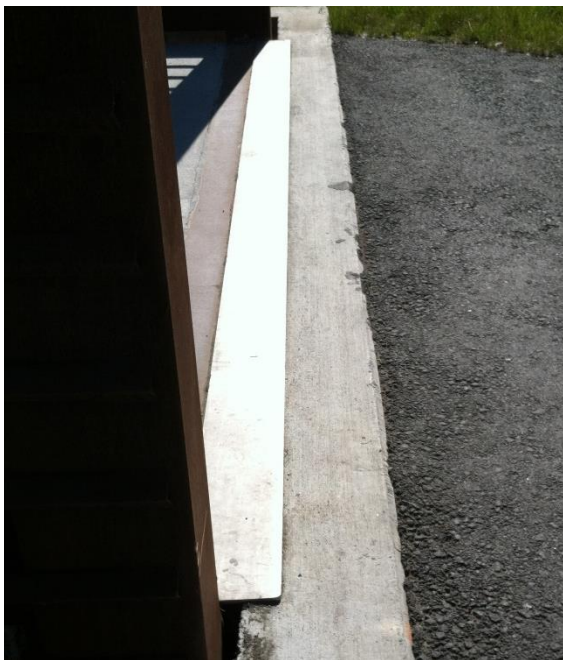
Figure 12. Covered Expansion Joint
