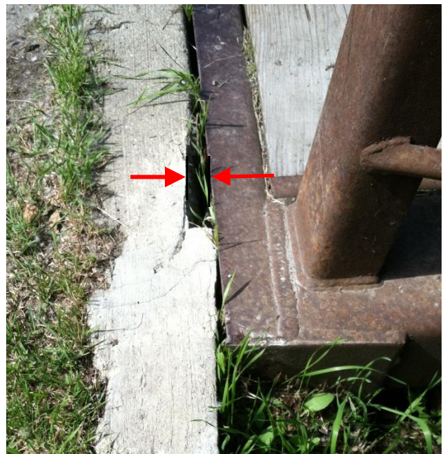
Figure 13. Expansion Joint Gap
