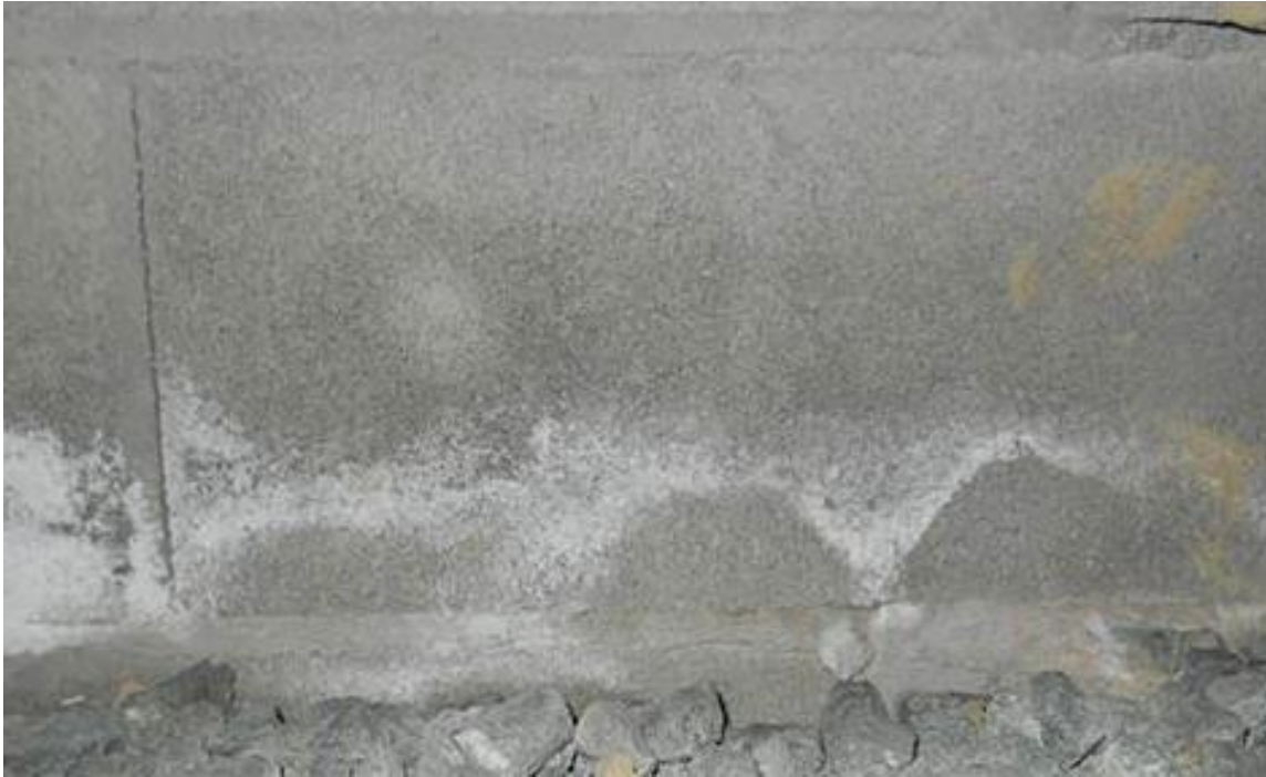
Figure 21. Concrete Efflorescence
