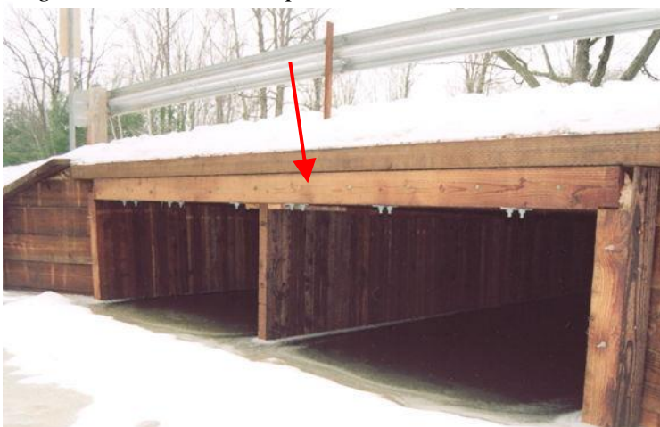
Figure 23. Timber Parapet
