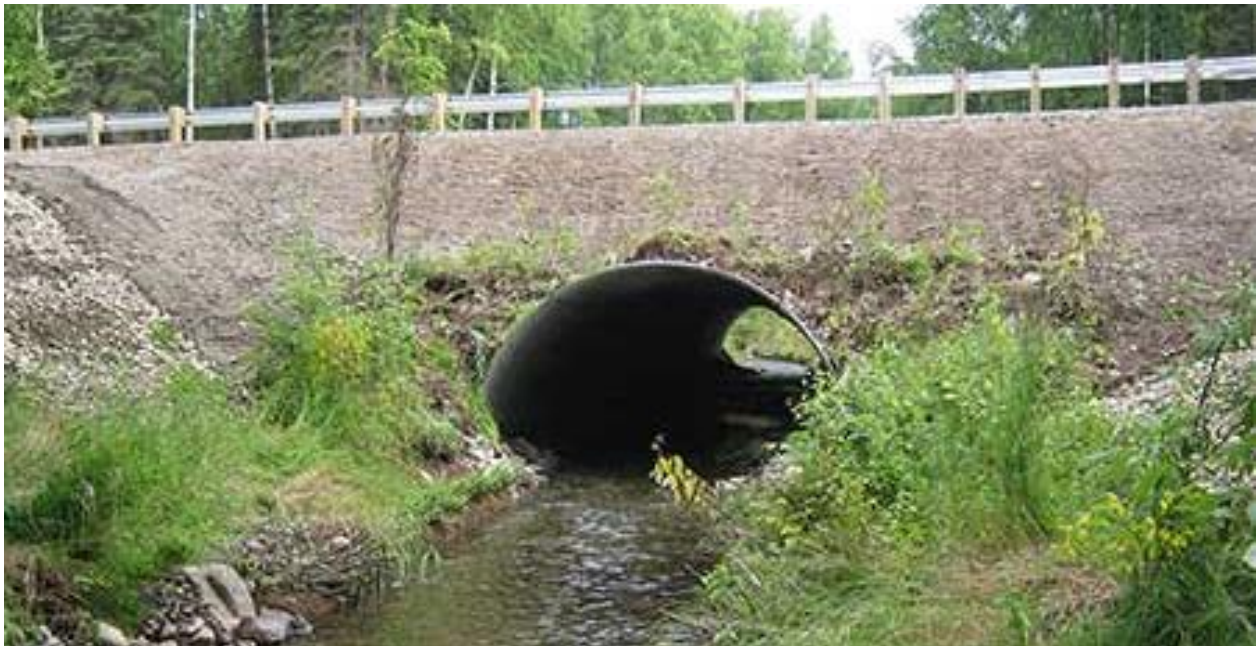
Figure 4. Type C Bridge
