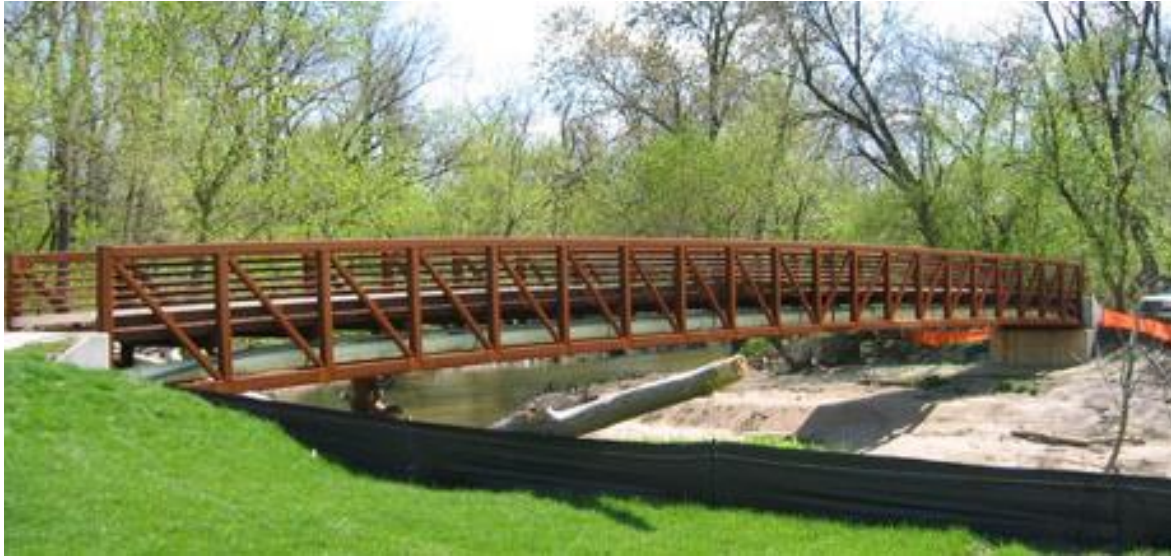
Figure 3. Type B Bridge
