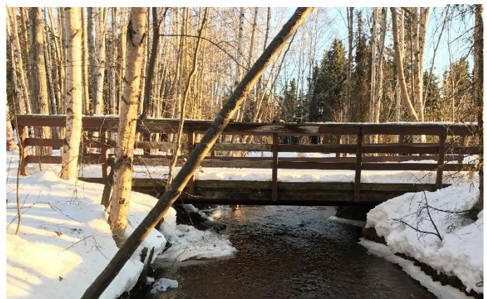
Figure 7. Type D Bridge
