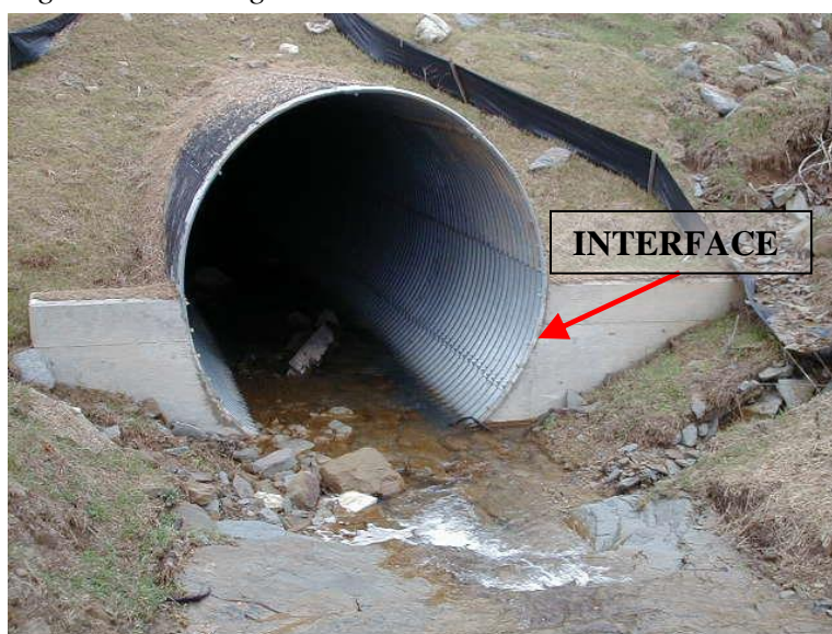
Figure 26. Corrugated Steel Culvert
