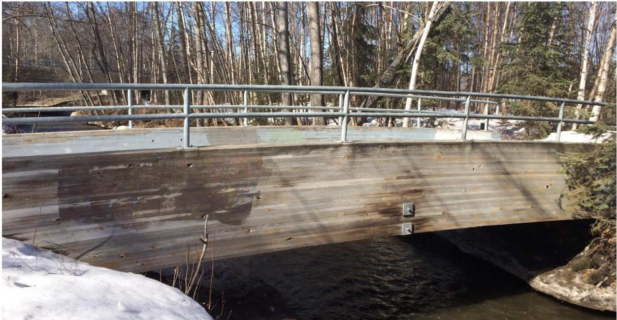
Figure 5. Type D Bridge
