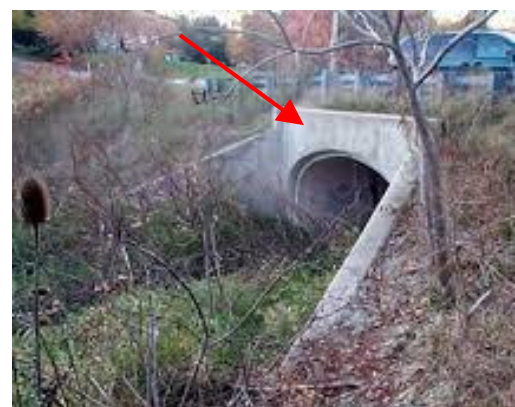
Figure 24. Concrete Parapet
