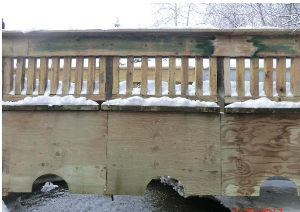
Figure 6. Type D Bridge
