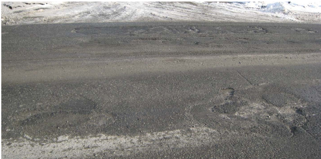
Figure 19 Settlement failure due to subsurface saturation and frost action.
